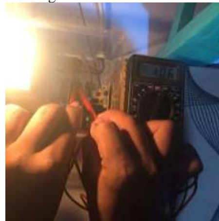
Fig. 12 Measurement Using Multitester on AC Light Dimmer Module
